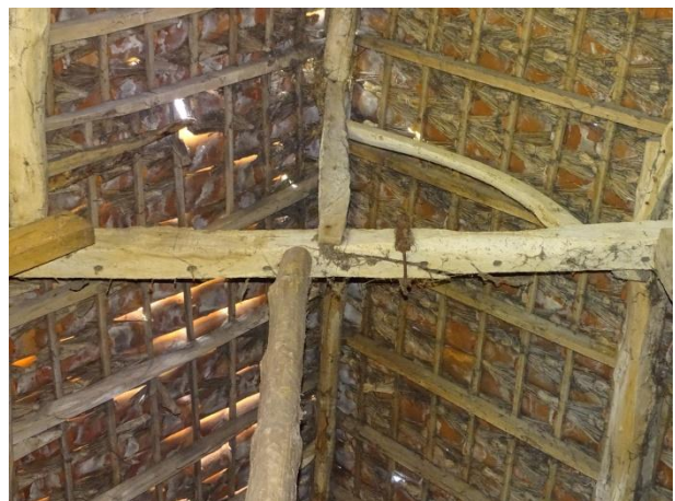
Afb. 3.125 Sporen in ankerbalk in spant 1
