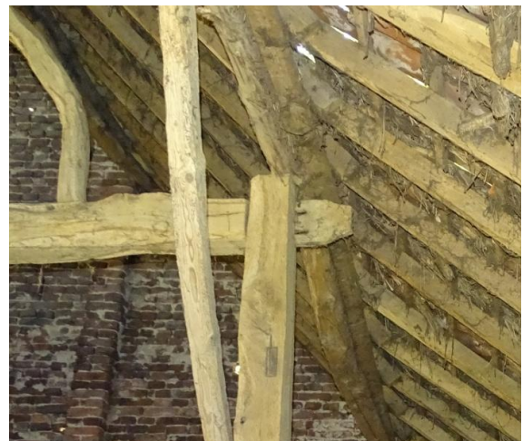
Afb. 3.124 Detail ankerbalk spant 1
