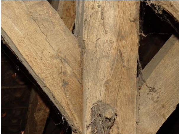
Afb. 3.106 Detail nokgordingschoor
